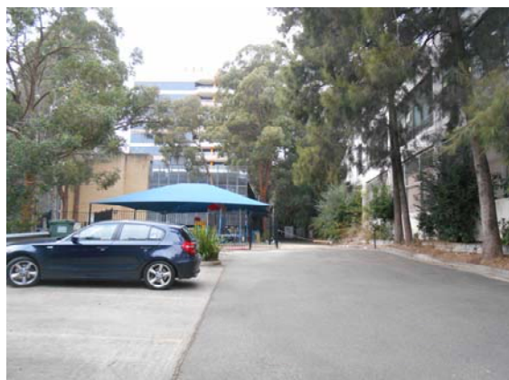
Photograph 6: View of ground level carpark located to the west of the Childcare Centre, 18-20 Orion Road (June 2015)
