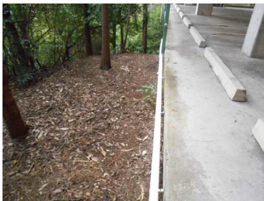
Photograph 11: PVC pipe running west-east along the northern edge of the carpark, 18-20 Orion Road (June 2015)
