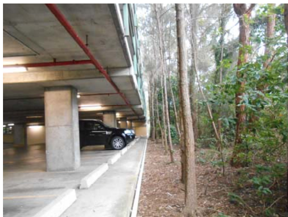
Photograph 12: view of bush strip to the north of the carpark, 18-20 Orion Road (June 2015)
