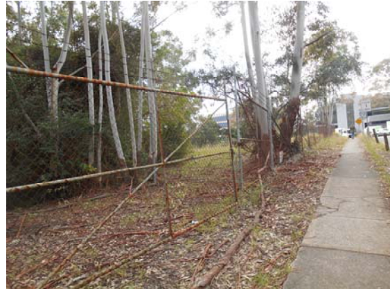
Photograph 24: View of fence along the southern boundary of 14-16 Orion Road (June 2015)
