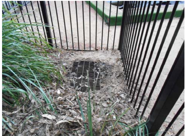
Photograph 18: View of stormwater/drain system at the vicinity of the Childcare Centre, 18-20 Orion Road (June 2015)
