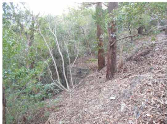
Photograph 4: View of sandstone brick square-shaped structure and associated pipe located to the north of the access road at 18-20 Orion Road (June 2015)
