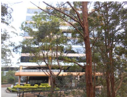
Photograph 3: View of multilevel building on 18-20 Orion Road (June 2015)
