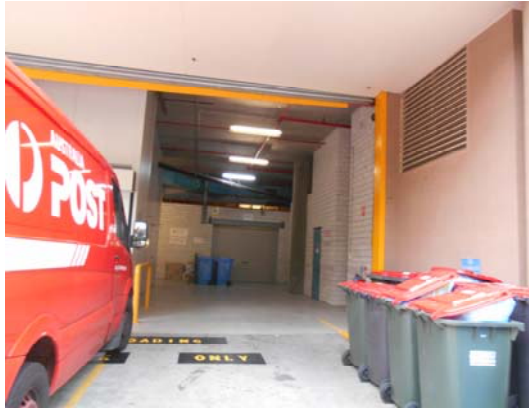
Photograph 7: View of loading dock and waste facility located at the southern end of the multilevel building, 18-20 Orion Road (June 2015)
