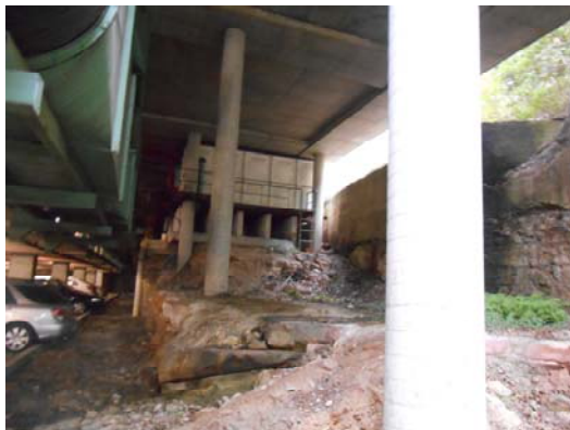
Photograph 15: view of the squared-shaped water tank located underneath the building footprint (right) and the carpark exhaust pipe system (left), 18-20 Orion Road (June 2015)
