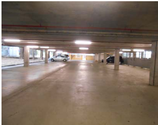
Photograph 13: View towards the east end of the carpark, showing Childcare Centre at the end, electrical substation to the far left, 18-20 Orion Road (June 2015)
